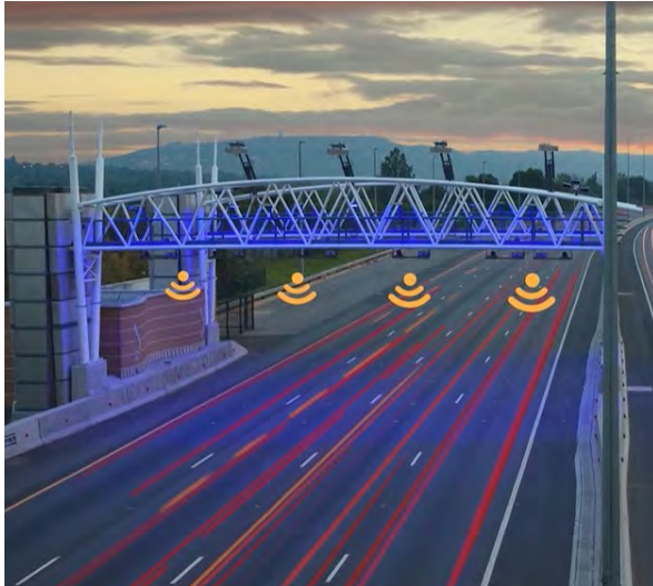
Figure 1-2. Electronic Toll Collection System
