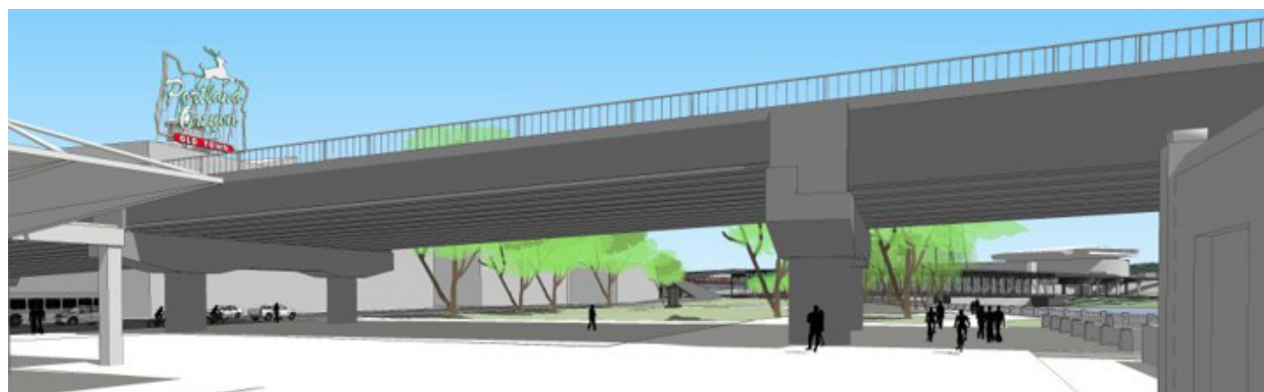
Rendering of girder structure type over Waterfront Park near downtown.
