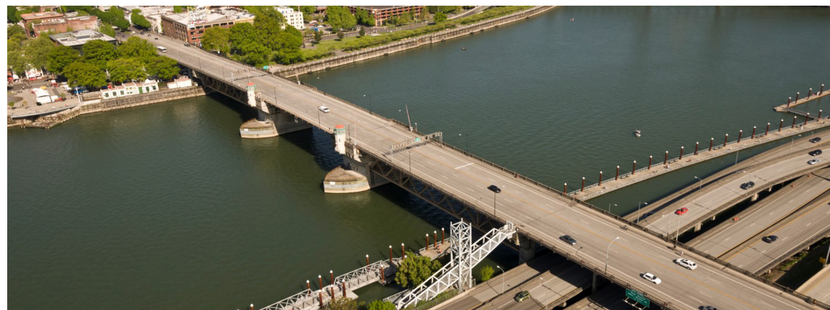
Aerial view of the existing Burnside Bridge looking northwest towards Old Town Chinatown.
