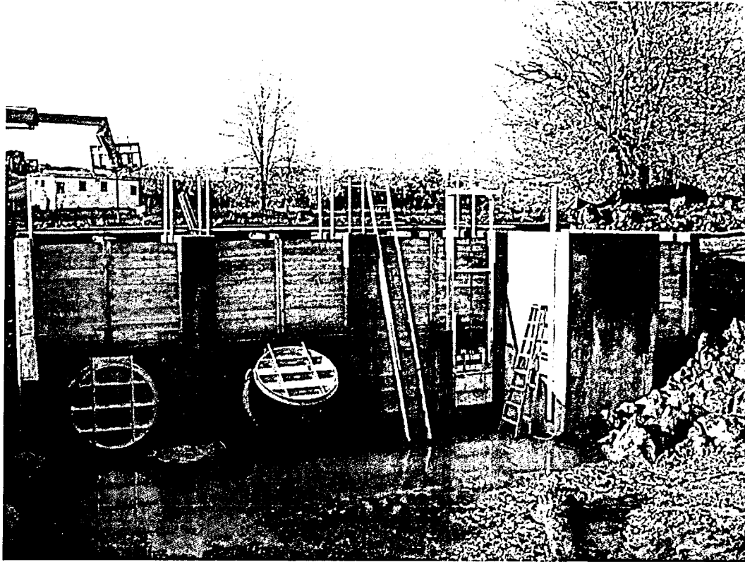
Figure 3: Water Control Structure.
