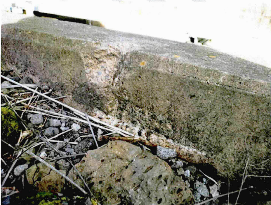
Photo A6: Spall in Northeast Wall
