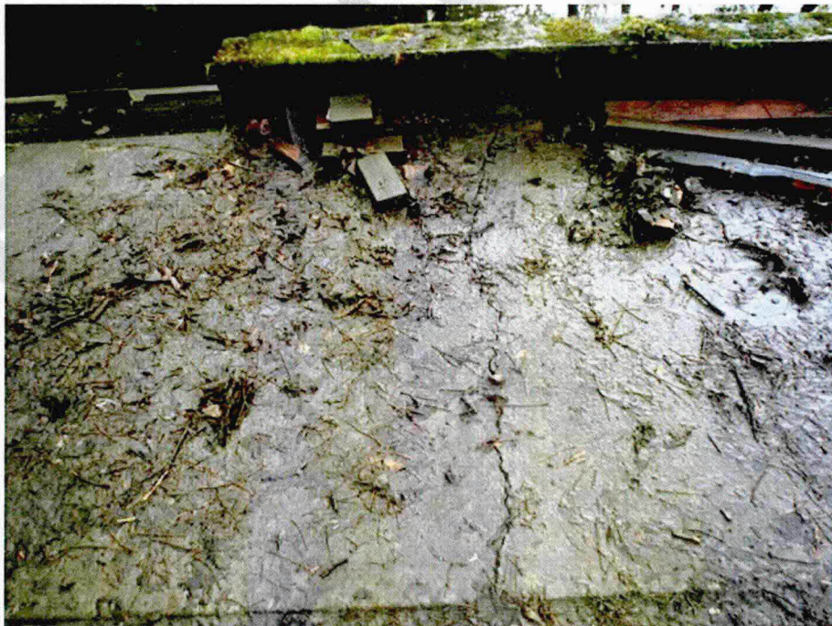
Photo A50: Crack in Slab-On-Grade
