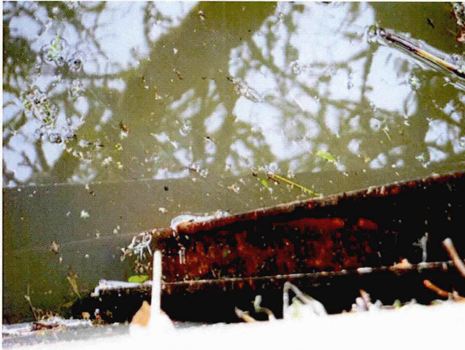
Photo A55: Typical Corrosion on Miscellaneous Metal Framing
