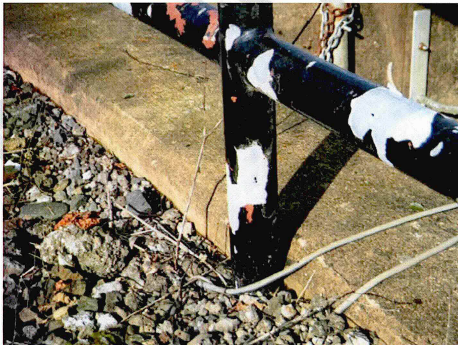
Photo A10: Northeast Wall – Typical Buried Rail Post
