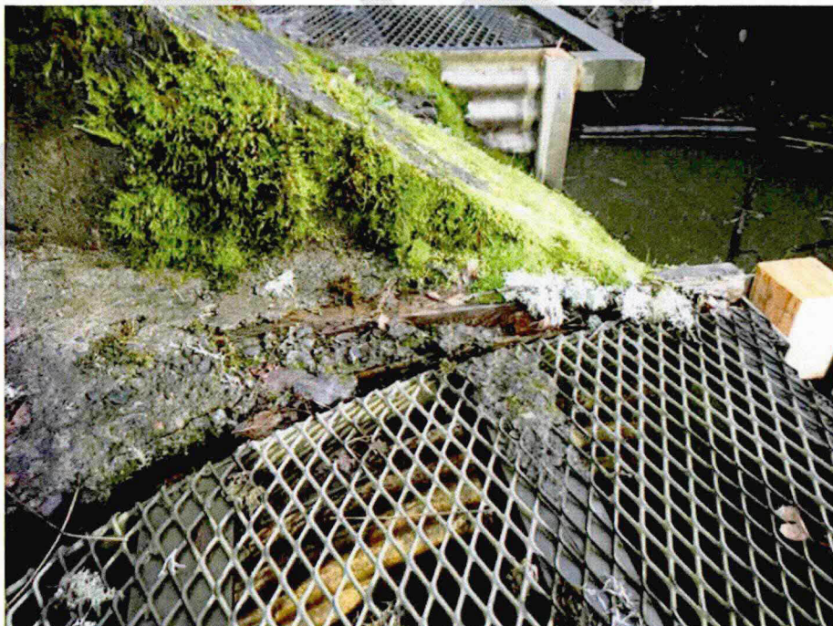
Photo A56: Inset Wood and Gap at Inlet
