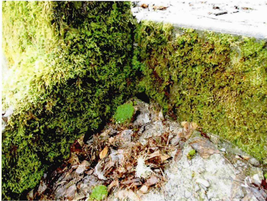
Photo A47: South Face – Void at Base of Slab-On-Grade Near Headwall
