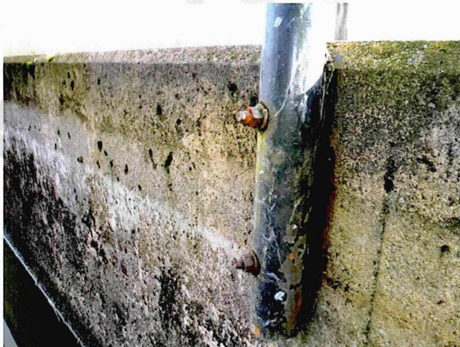
Photo A12: Typical Rail Post Connection – Corrosion at Anchors
