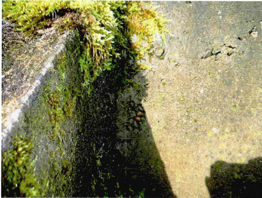
Photo A51: Rock Pocket in Headwall
