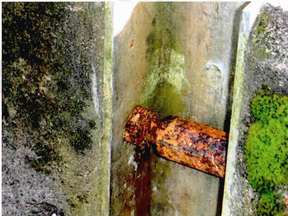
Photo A20: Pin Corrosion at Inlet Keeper Slots
