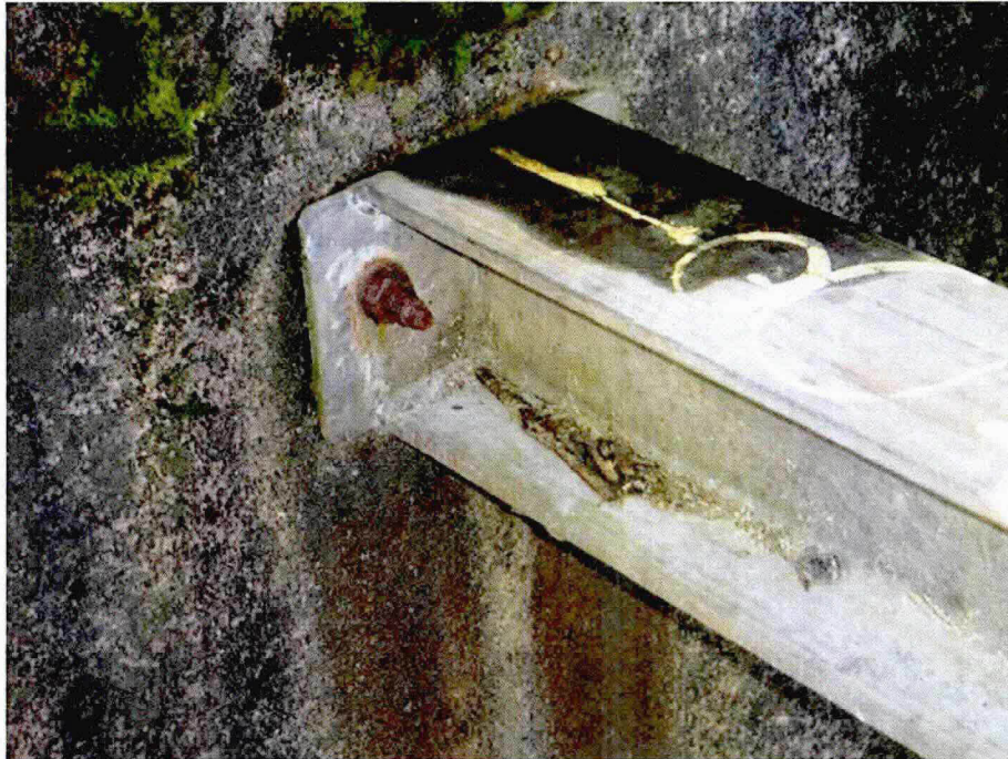
Photo A23: Typical Corrosion on Miscellaneous Metal Framing
