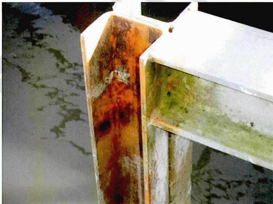
Photo A22: Typical Corrosion on Miscellaneous Metal Framing
