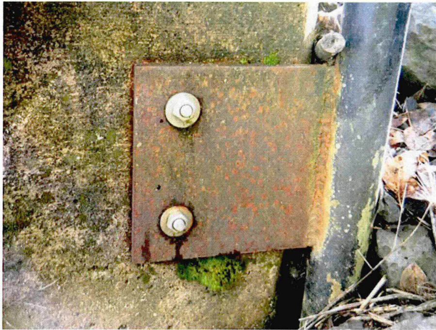
Photo A9: Northern End of Northeast Wall – Rail Post Connection
