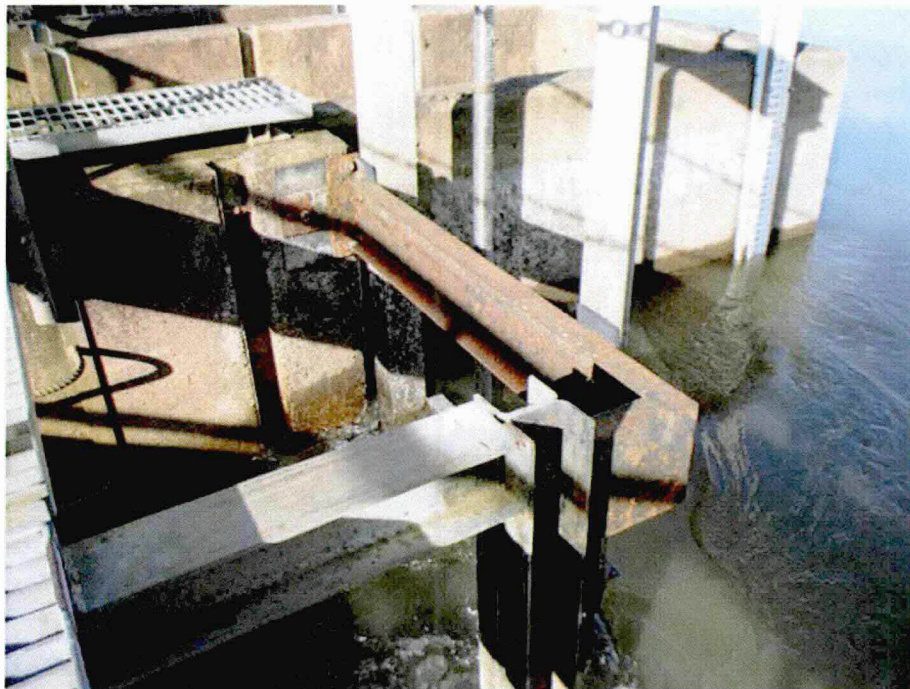
Photo A21: Typical Corrosion on Miscellaneous Metal Framing
