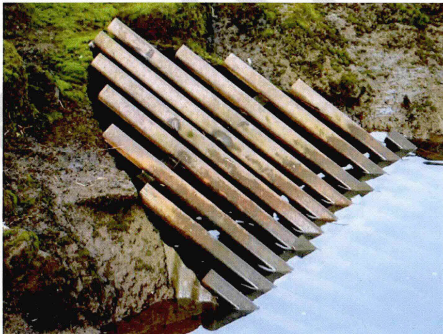
Photo A30: Typical Steel Outlet Screen
