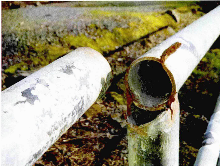
Photo A15: Southwest Wall – Separated Top Rail
