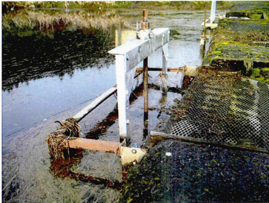
Photo A31: Typical Corrosion on Miscellaneous Metal Framing
