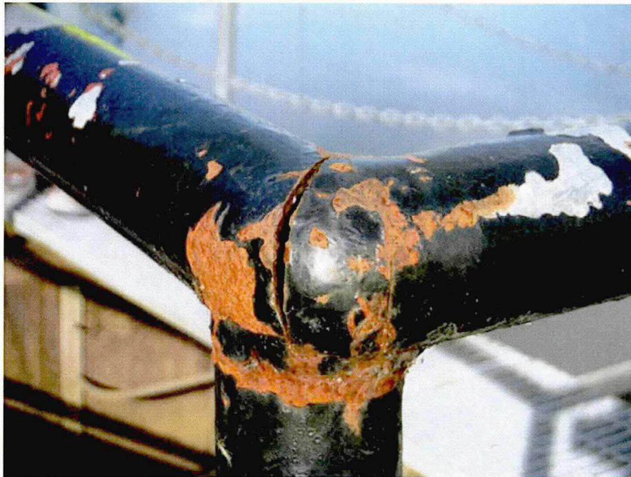
Photo A13: Southern End Northeast Wall – Split Top Rail
