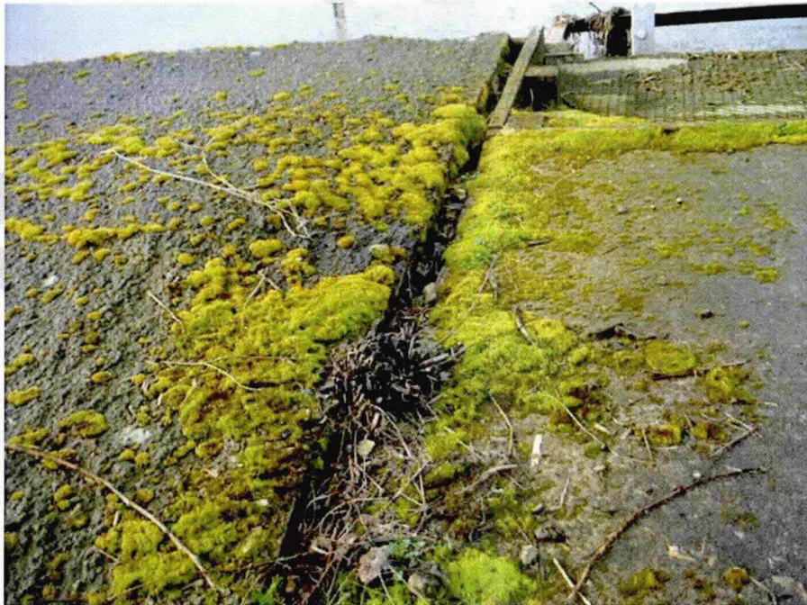
Photo A36: South Inlet – Deteriorated Wood
