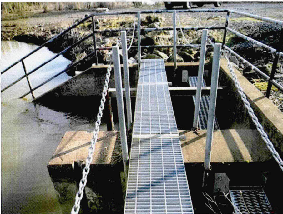
Photo A18: Walkway Over Inlets and Chain Railing
