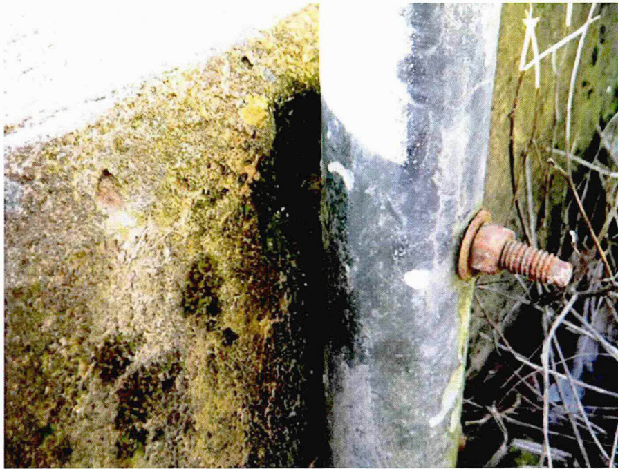
Photo A7: Spall in Southwest Wall at Rail Post Anchor
