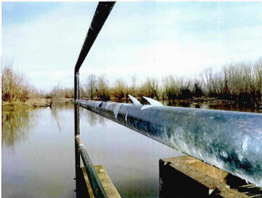
Photo A16: Typical Railing – Coating Loss and Peeling
