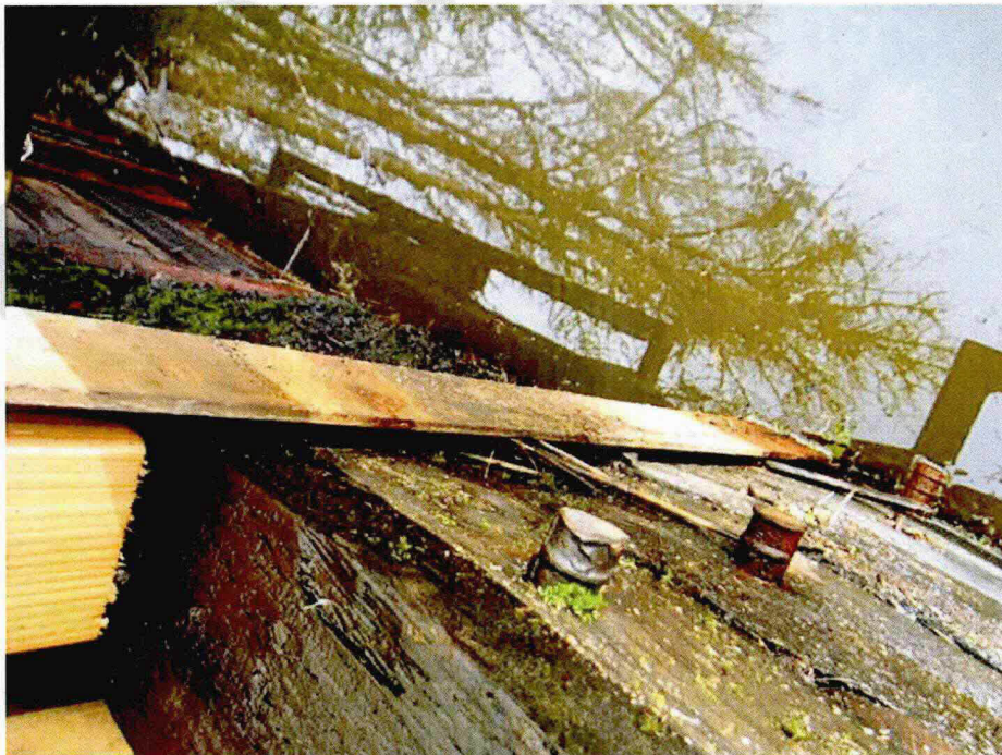
Photo A54: Typical Corrosion on Miscellaneous Metal Framing
