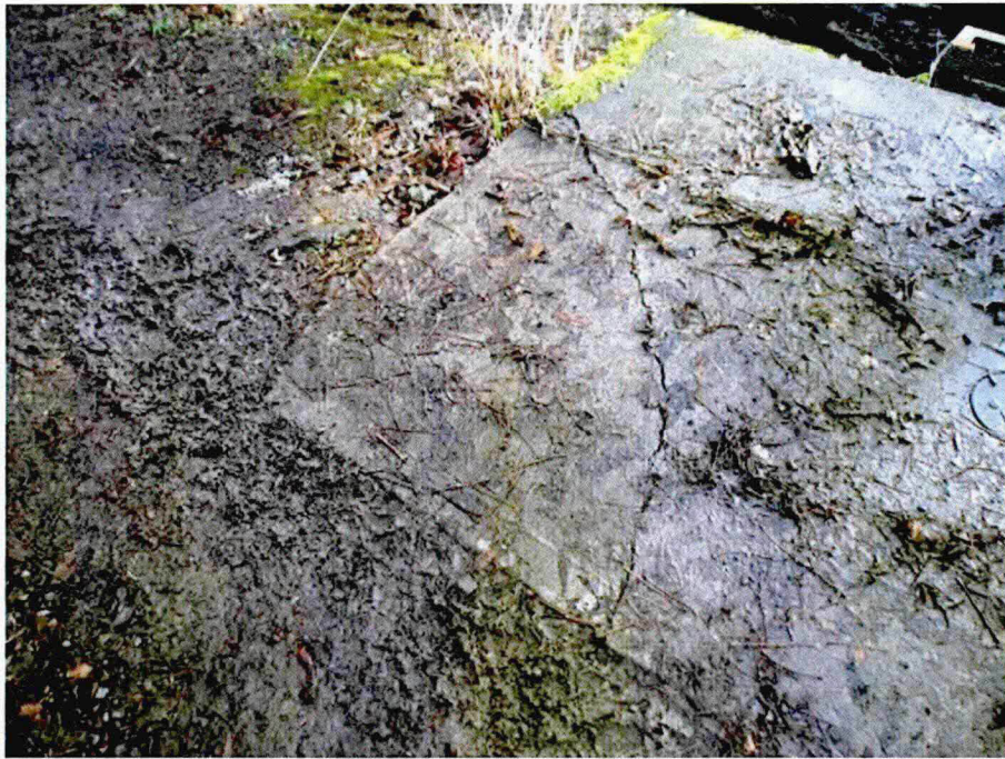
Photo A49: Crack at Corner of Slab-On-Grade
