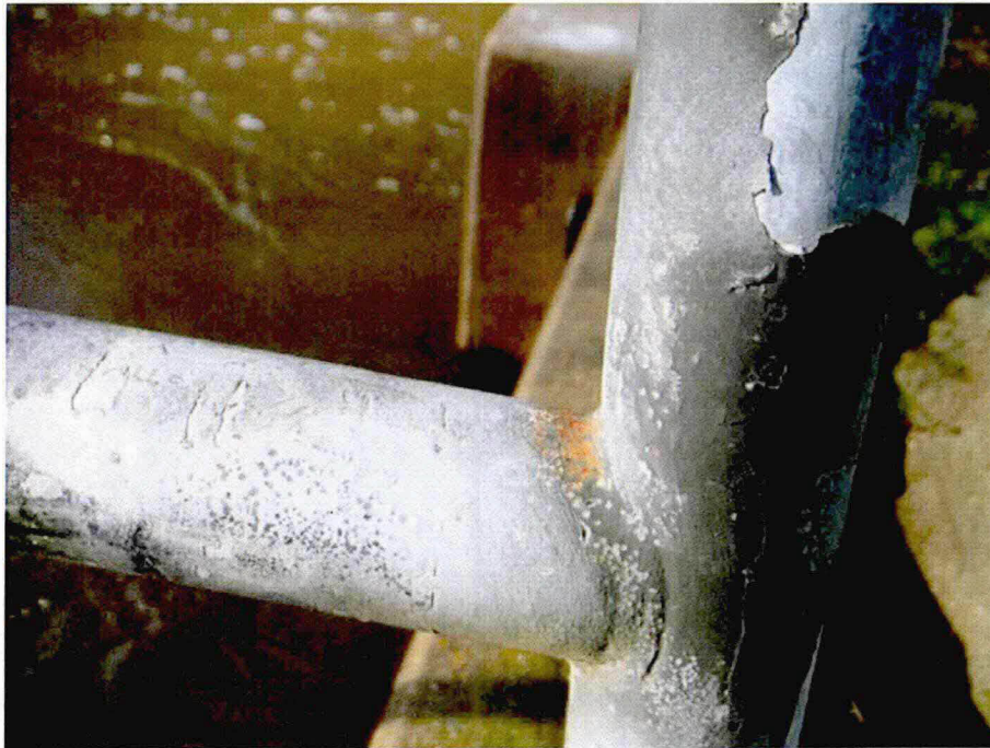
Photo A17: Typical Railing Corrosion
