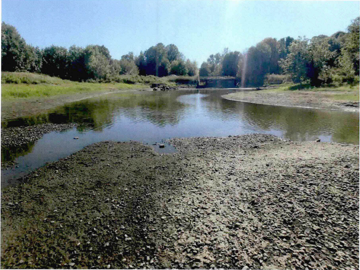
Photo 1: Channel upstream of Water Control Structure, approximately station 2+00 (August 15, 2016)
