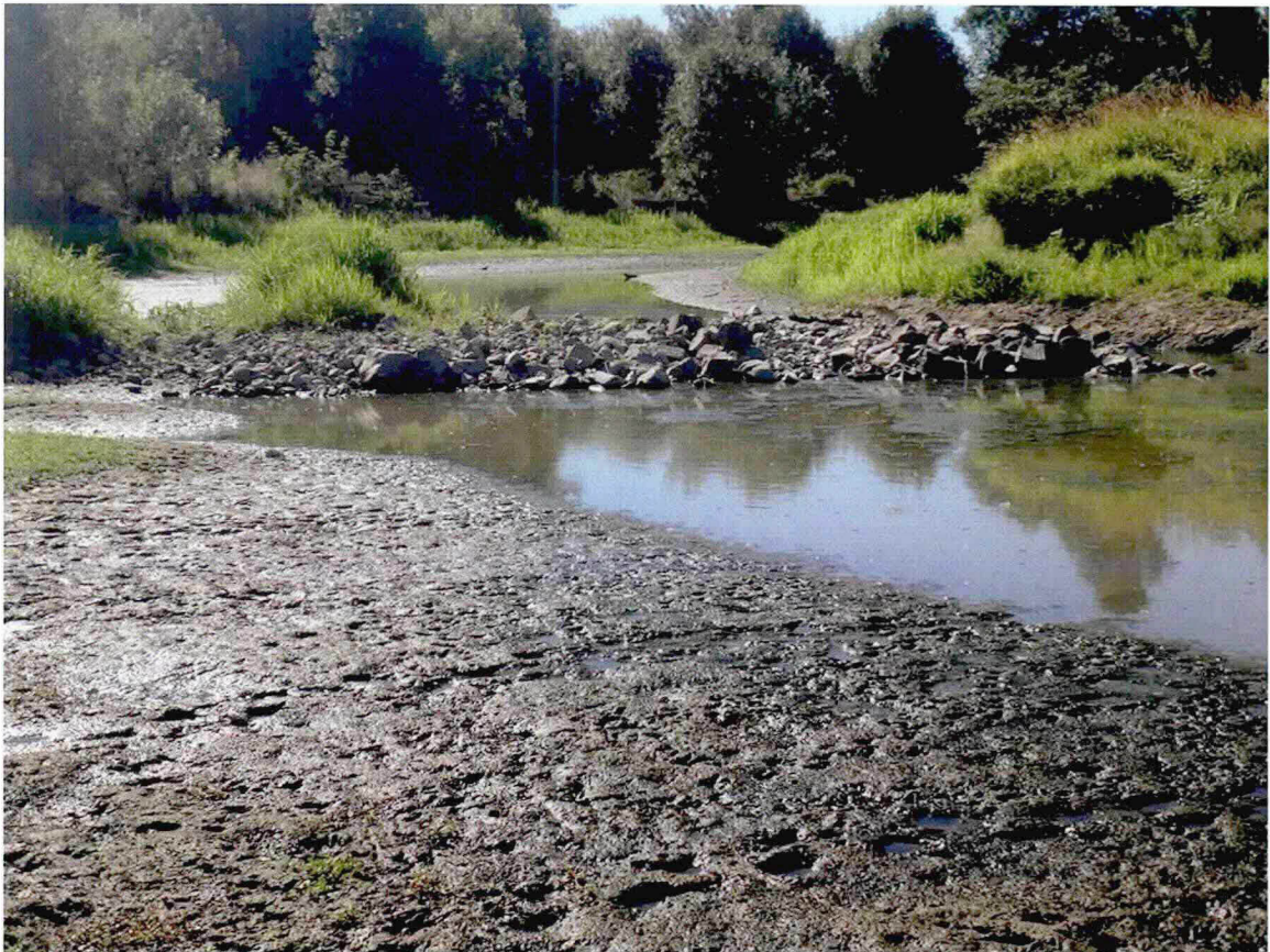
Photo 2: Existing Derelict Road Crossing (August 15, 2016)
