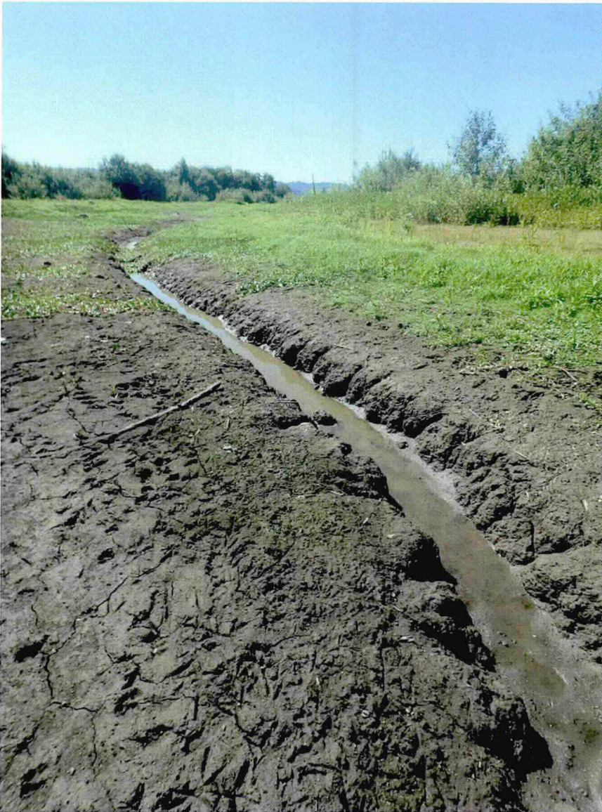
Photo 5: Existing channel at approx. station 44+00, looking towards lake (August 15, 2016)
