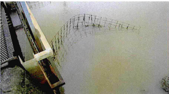
Reanchor debris rack on NWCS
