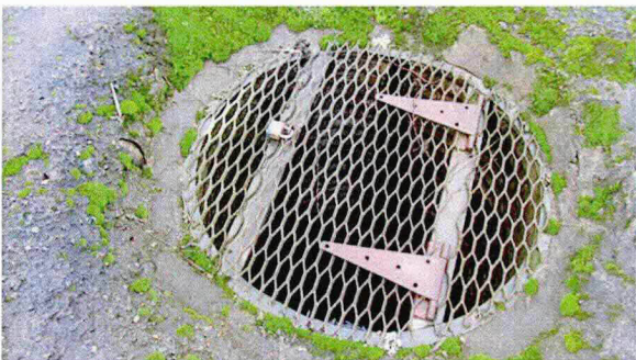
Load boards into central riser in NWCS
