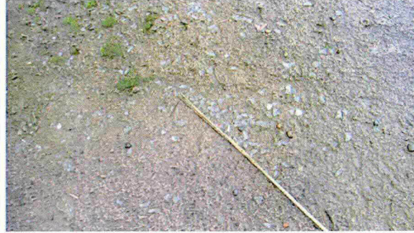
Broken glass on NWCS
