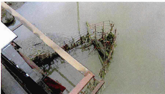
Clean out debris from NWCS
