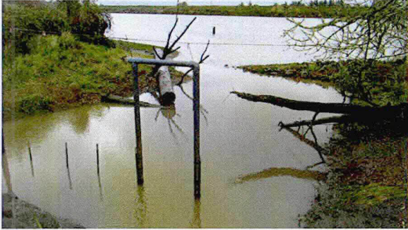
Repair downstream boom at NWCS
