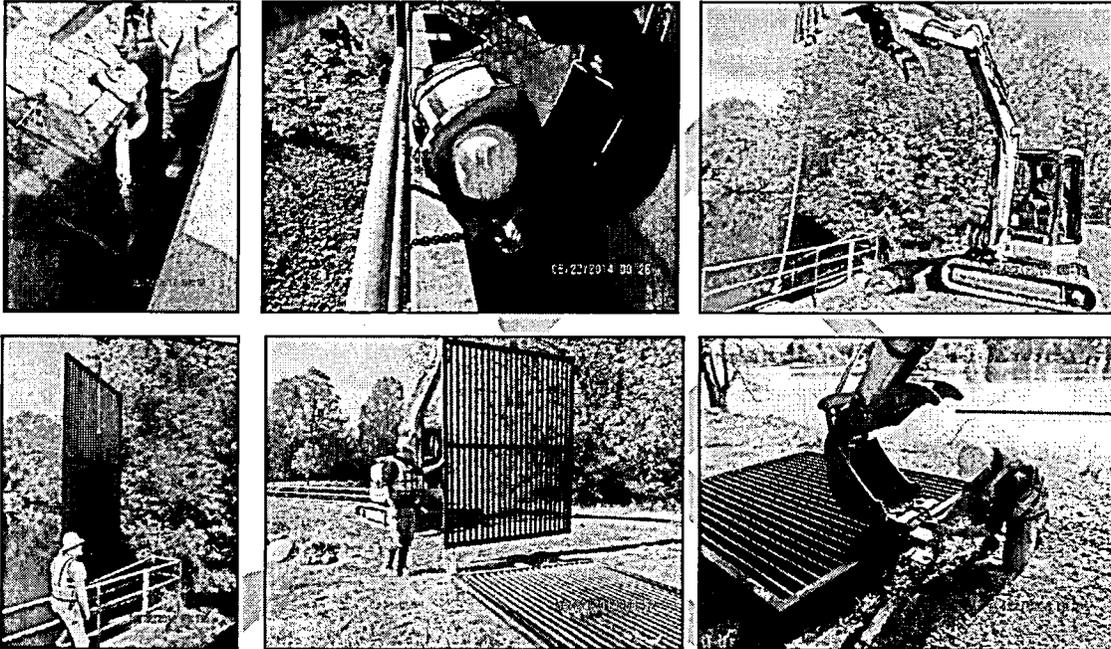
**Fall board installation (late Oct/early Nov - by Veterans Day – at Scientist Confirmation).** Install trash racks to prevent logs and debris from entering the bays. Before racks go in, walk in the bays to make sure there are no logs or debris in structure and lube gaskets etc. See if it's possible to cut out the bottom boards that may be stuck there.
