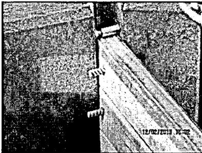
Rebar picks should be on each board. Use 5/8" rebar – drill hole through and pound in. Cut rebar to 6" length and grind off ends.
