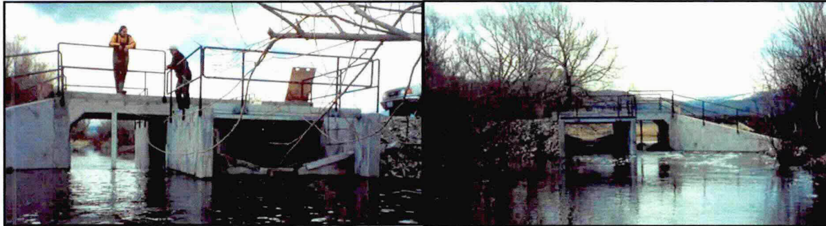
Figure 30. Pool-weir-chute water-control structure on Ladd Creek. Left photo: looking downstream (emergency spillway on left, and fish ladder on right). Right photo: looking upstream.
