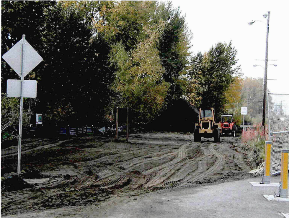
Figure 3. View of old parking lot as new soil is added.
