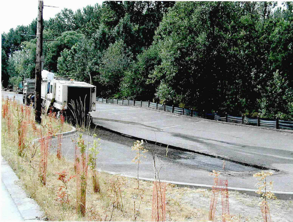
Figure 1. Removing asphalt from the old parking lot at Smith-Bybee.
