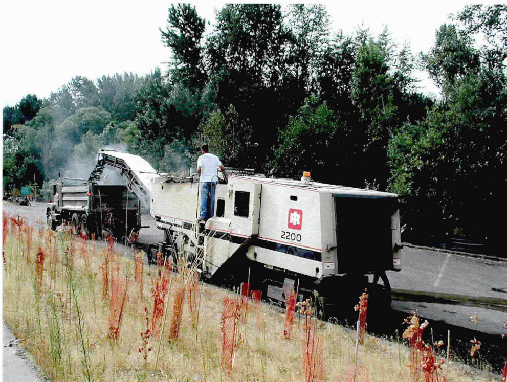
Figure 2. Another view of asphalt removal; the asphalt was recycled.
