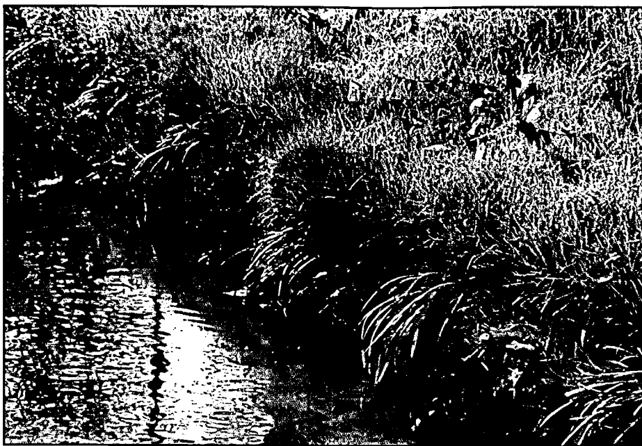
Live stakes of purple winter creeper, plugs of liriope and english ivy and grass, roots into the socks and into the banks.
