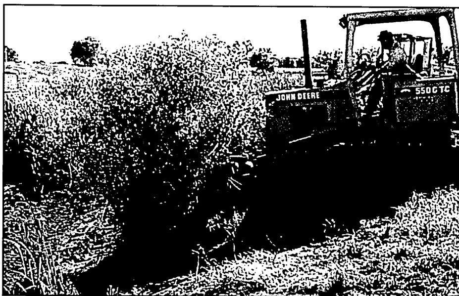
Bulldozer removing willow tree from PVC liner.
