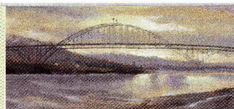
The 902-foot long center span of the Fremont Bridge was jacked 175 feet into place in 1973 over a 50-hour period. It is the world's longest tied-arch orthotropic deck bridge without piers in the main channel.
