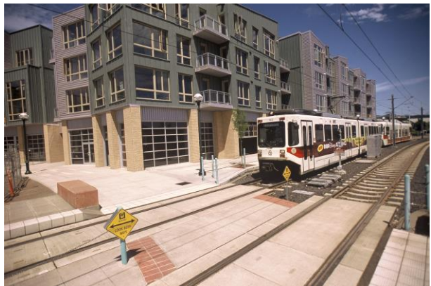
TriMet MAX train along Transit Oriented Development (TOD) project Photo courtesy of TriMet
