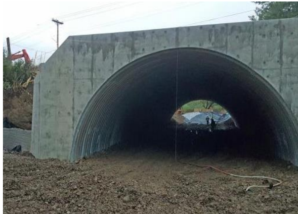
Stark Street Beaver Creek Culvert Replacement Photo courtesy of Multnomah County
