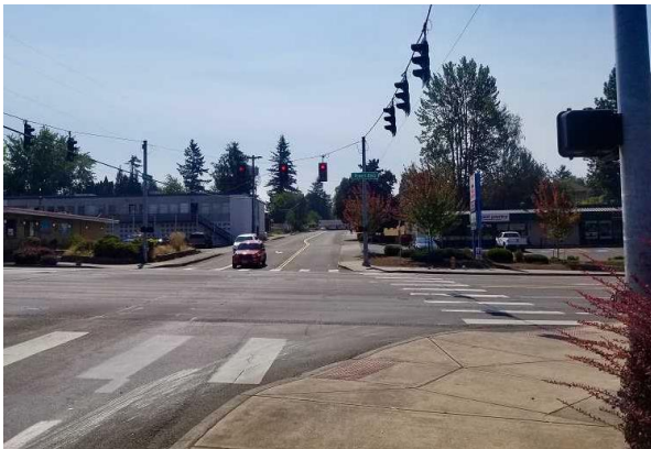
Existing Conditions on NE Cleveland Ave: Stark St to Powell Blvd Photo courtesy of Gresham
