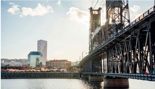
Steel Bridge connecting NE Portland to downtown Photo courtesy of ODOT
