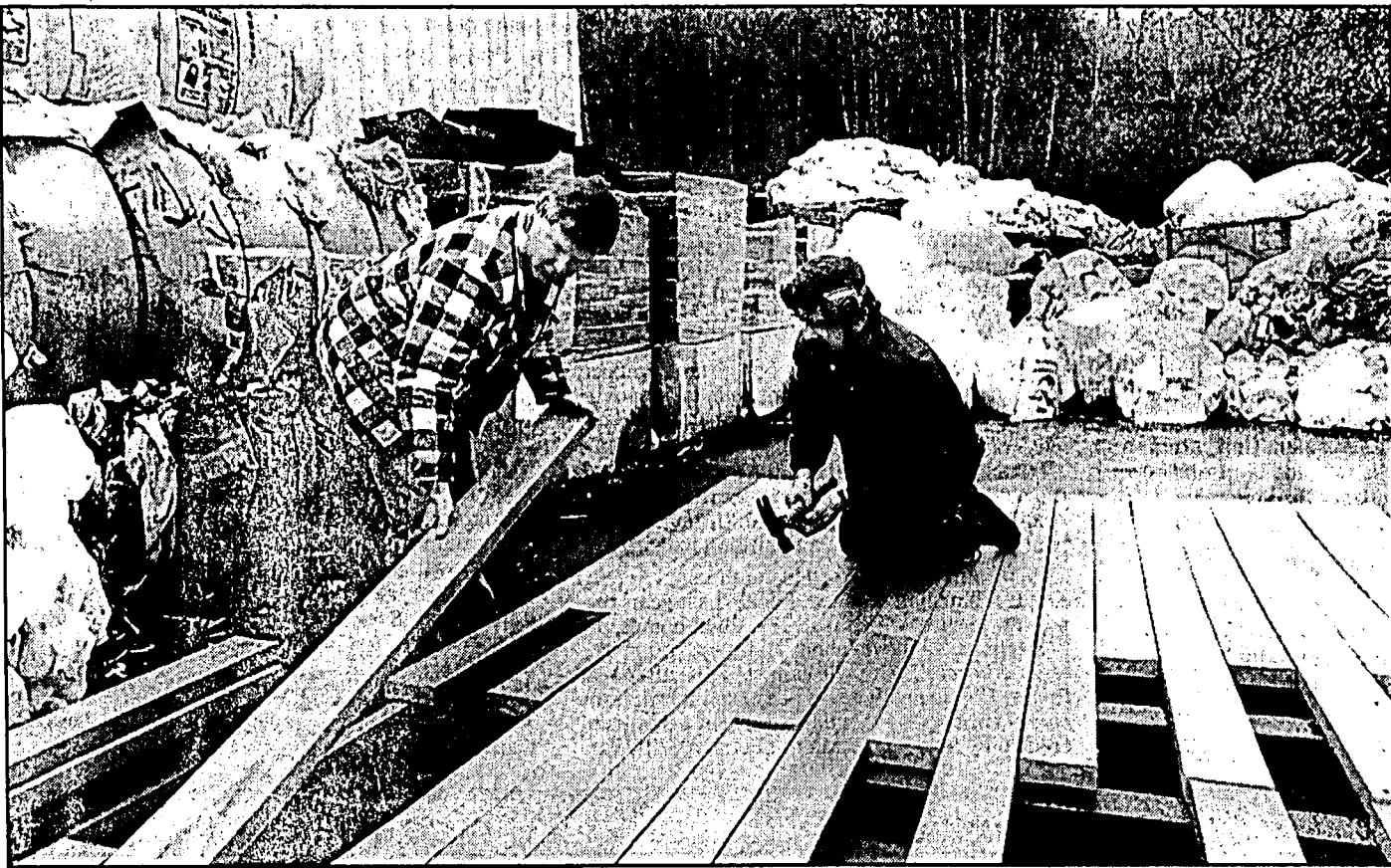
Above: Stan Kezar (left) and Gary Shipley build a deck using the plastic lumber made at Kezar's Enviro Lumber factory. Below: Shipley feeds waste plastic into a shredder at Enviro Lumber.
