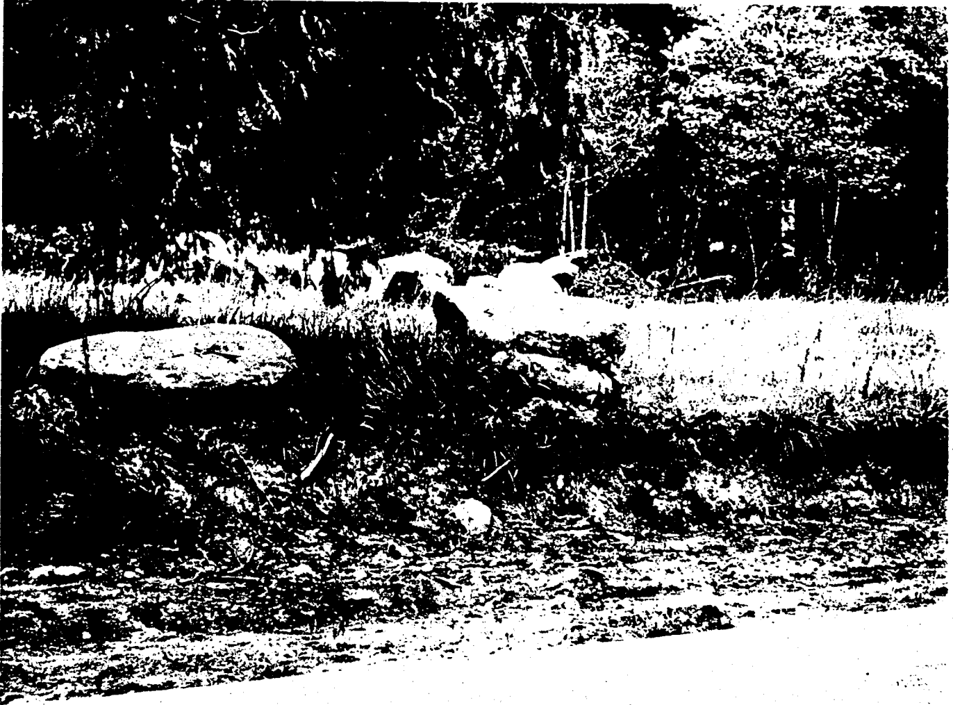
Figure 27.—Large stones and boulders excavated during street construction on Jory stony silt loam.
