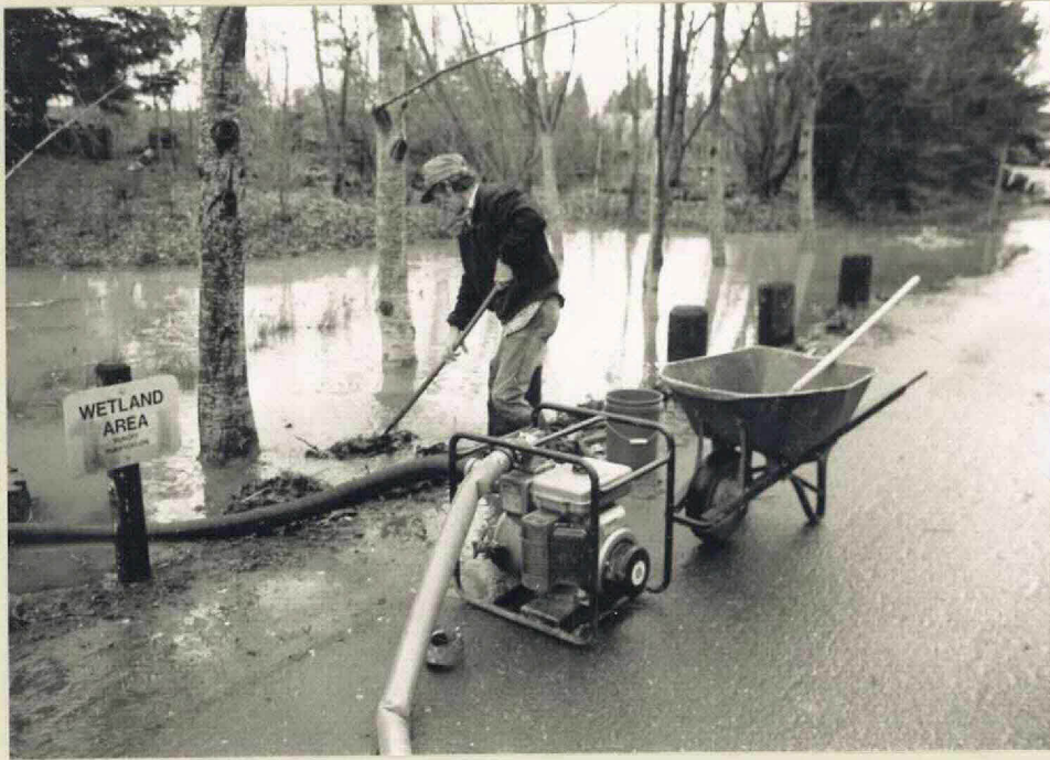
BASIN EXCAVATION USING RAKING & PUMPING TECHNIQUES
