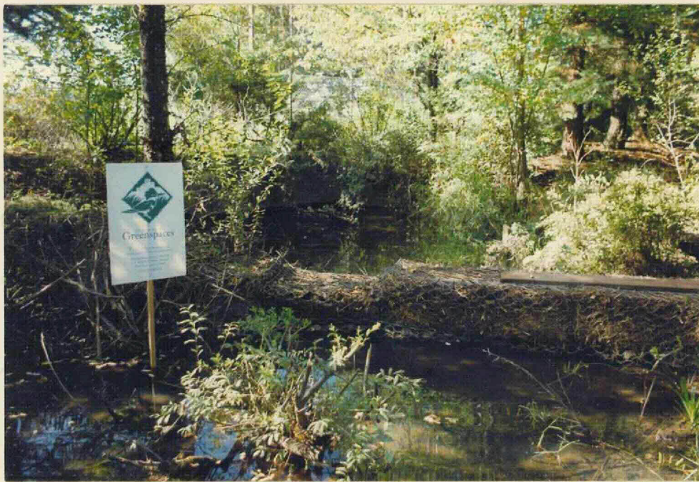
COMPLETED "PEOPLE MADE BEAVER DAM" FILTRATION WIER COMPLEX
