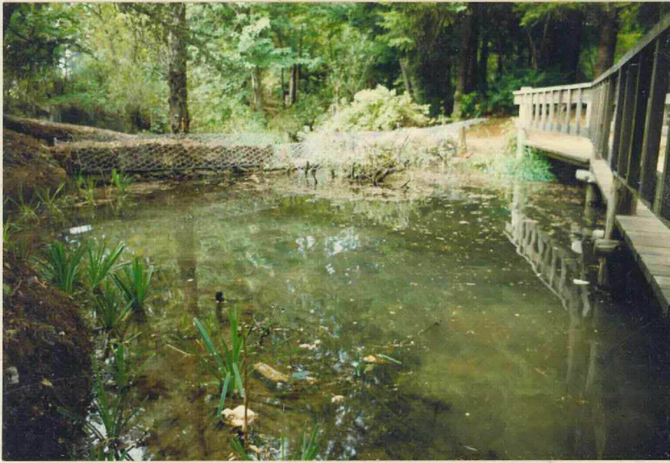
EXPANDED BIO-REMEDIATION BASIN WITH WIER & WALKWAY
