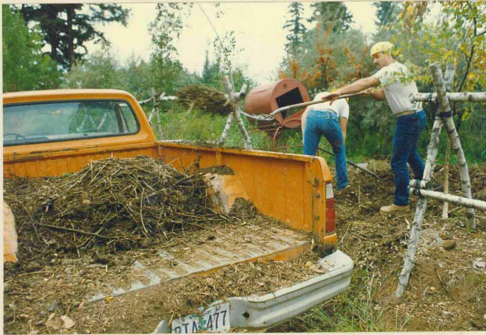
SITE PREPARATION FOR WETLAND BASINS (CORRECTIONS WORKERS)
