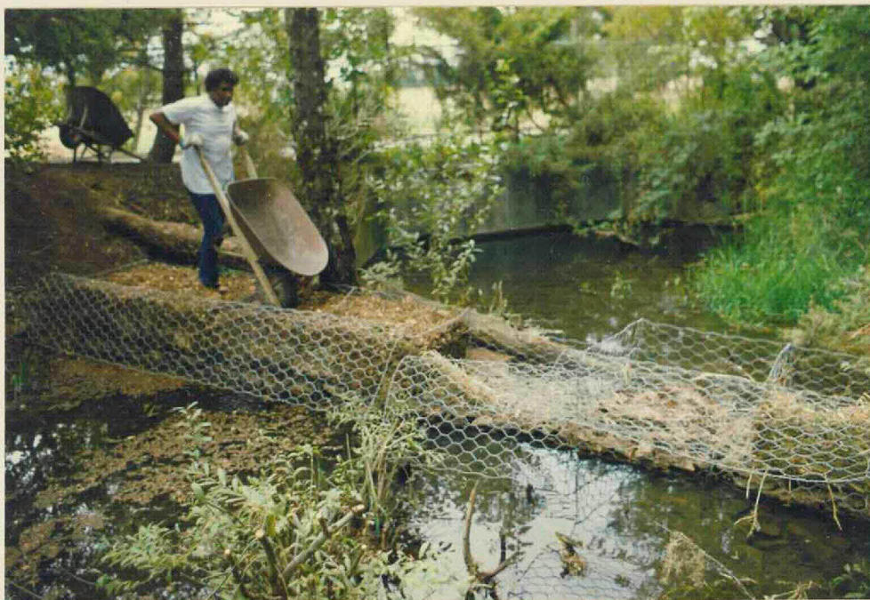
NEWELL CREEK HEADWATERS WIER CONSTRUCTION (CULVERTS VISIBLE)
