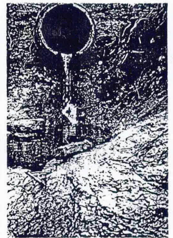
▲ EROSION UNDER A STORM WATER PIPE AT BINFORD LAKE.
