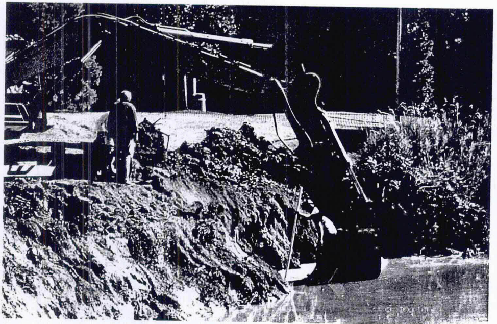
Toe of boulder terraced bank being installed two feet below stream bed.
