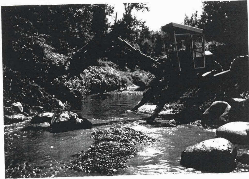
Spyderhoe placing boulders into stream bank.
