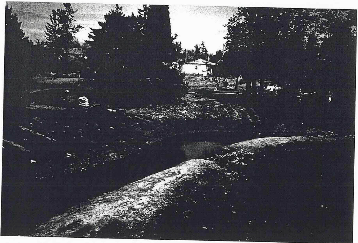
Completed bank stabilization and water quality pond prior to planting. May 2, 1997 site preparations for planting day.
