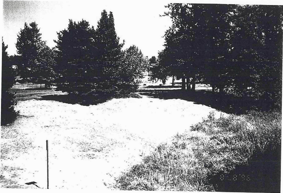
Water Quality Wetland Treatment Pond area before construction. Area is covered with large gravel which was a maintenance headache in addition to providing no habitat along the creek.
