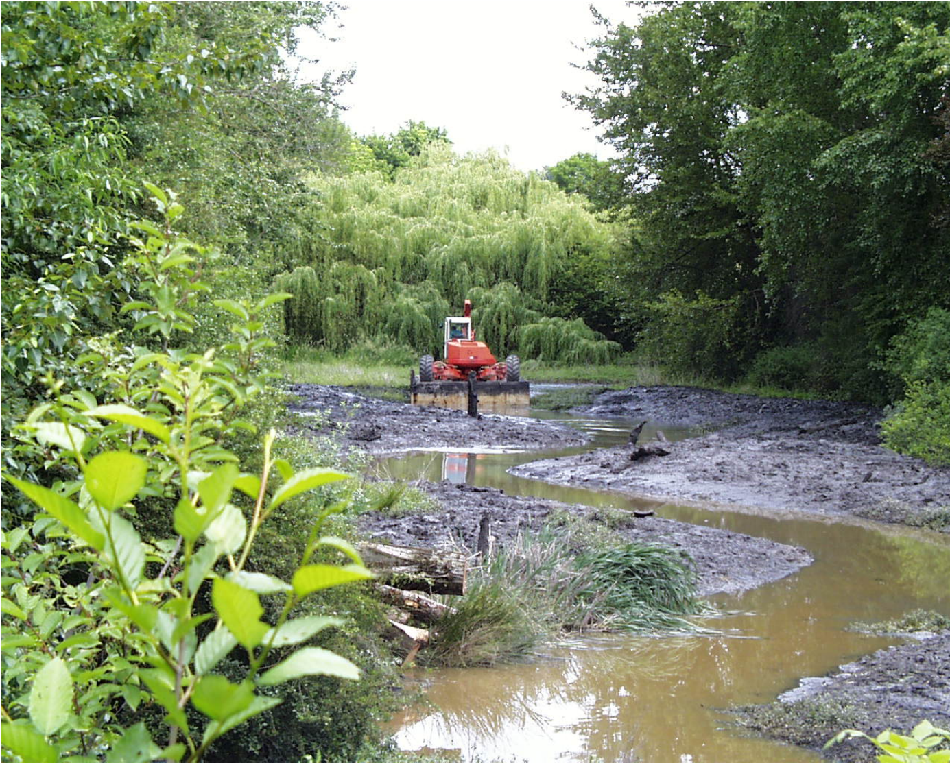
Multnomah County Drainage District's spiderhoe at work,2002..
