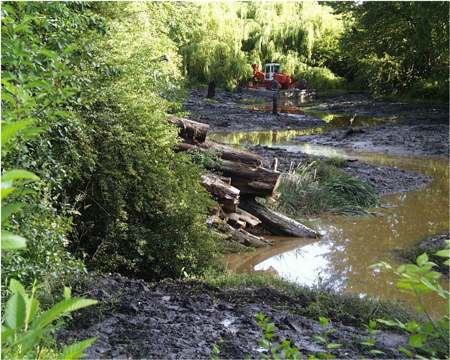
During reconstruction, the material removed from the channel was placed along the edges.
