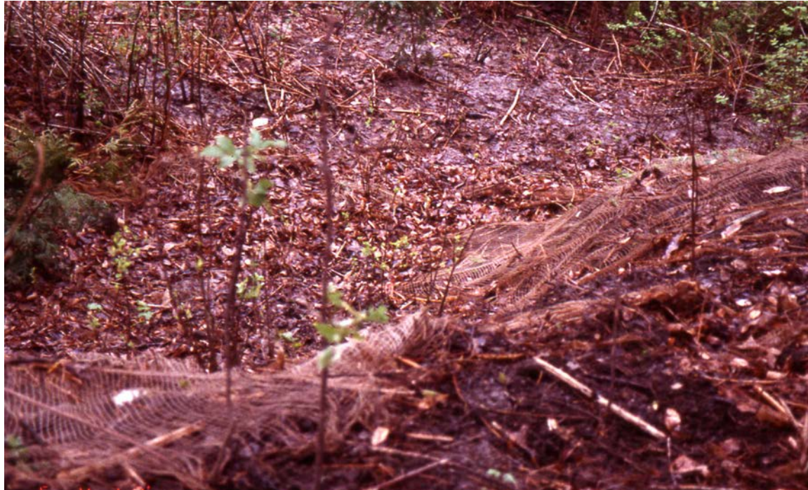
Erosion netting applied after removal of Blackberries on the stepper slope of Walker Slough in 1999.
