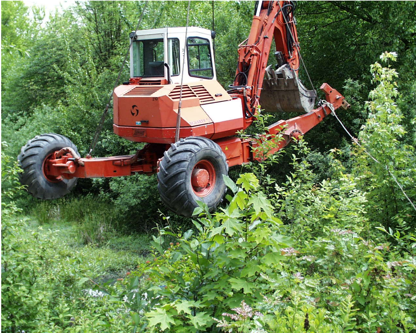
The spider hoe being lowered on to the barge.
