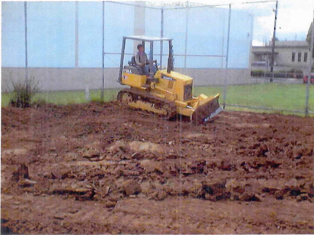
Grading after concrete removal
