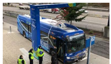
Beaverton Transit Center Overhead Pantograph Fast Chargers
