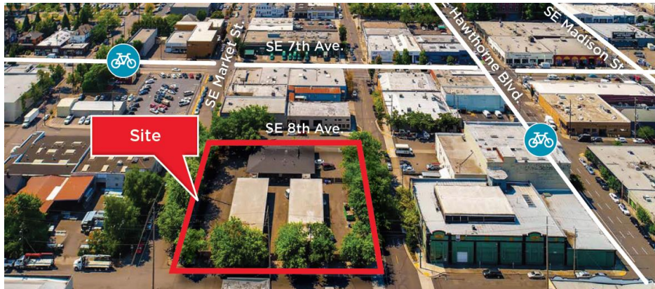
Figure 1. RID Deployment Center
