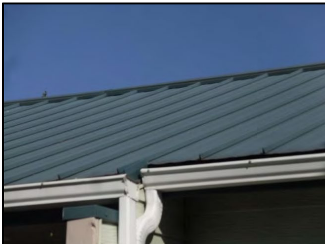
Typical roof drain gutters.
