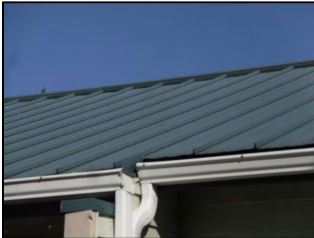
Typical roof drain gutters.
