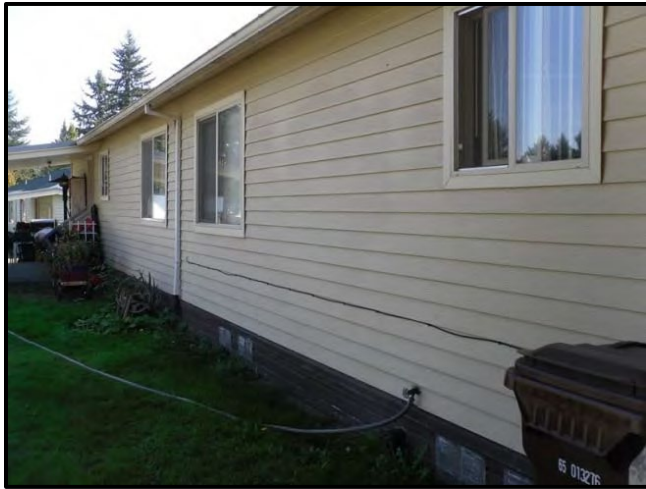
Typical apartment unit exterior wall finishes.
