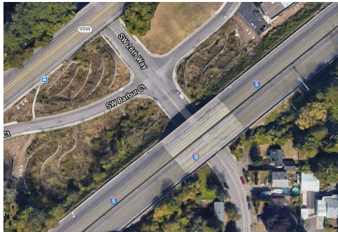
I-5 over 26 th Avenue Bridge Photo courtesy of ODOT
