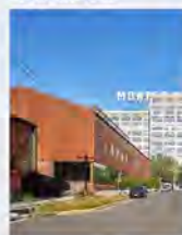
Development on NW Wilson which repurposed an existing industrial building with an updated form and new materials.
