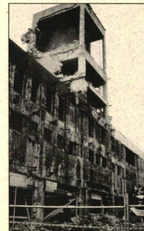
The Sears building structure was reused in Metro's renovation.
