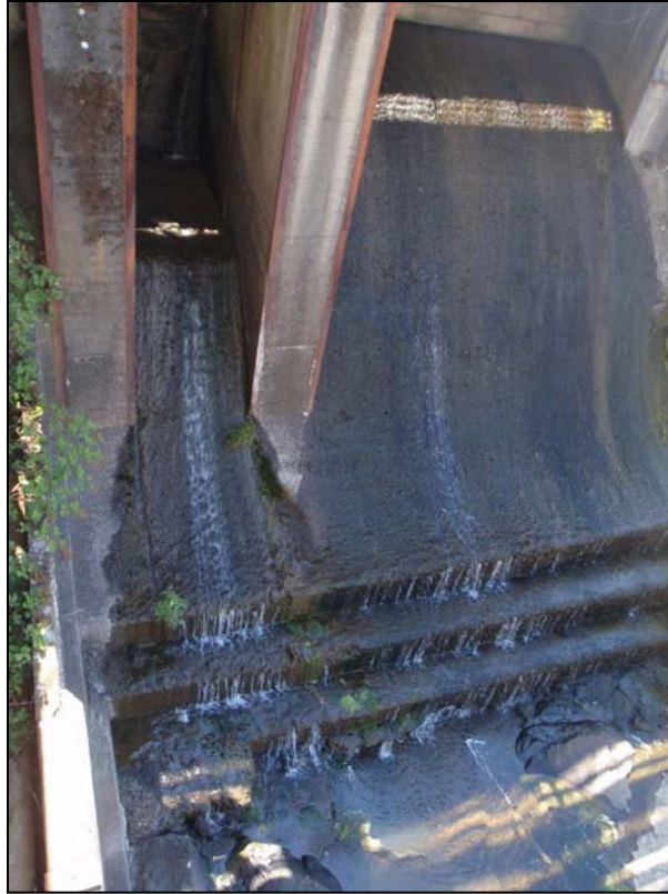
Photo 15. Flashboard weir on the PGE dam (08/03/2012).
