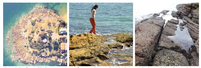
Figure 3, Sandstone blocks were extracted from on-site, weathered using water jetting, and placed around the margins of Barangaroo Reserve.
