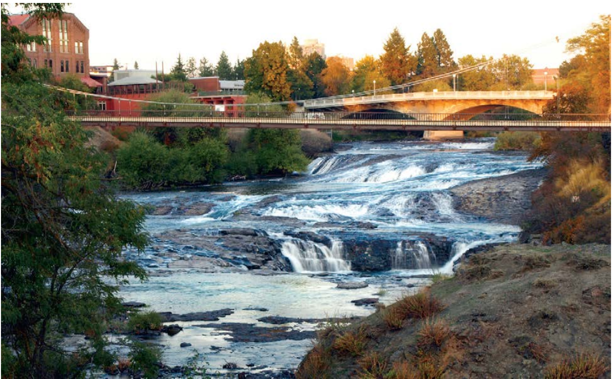
Figure 1, View of the Spokane River north channel after construction
