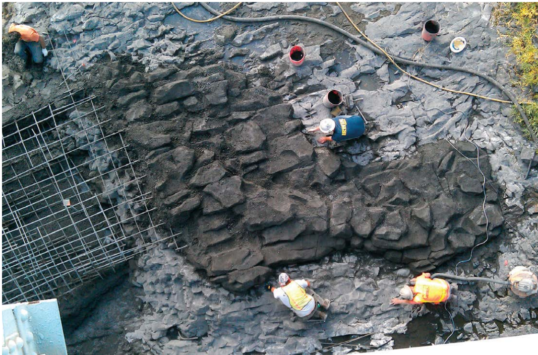
Figure 4, Construction workers sculpting concrete over a metal framework.
