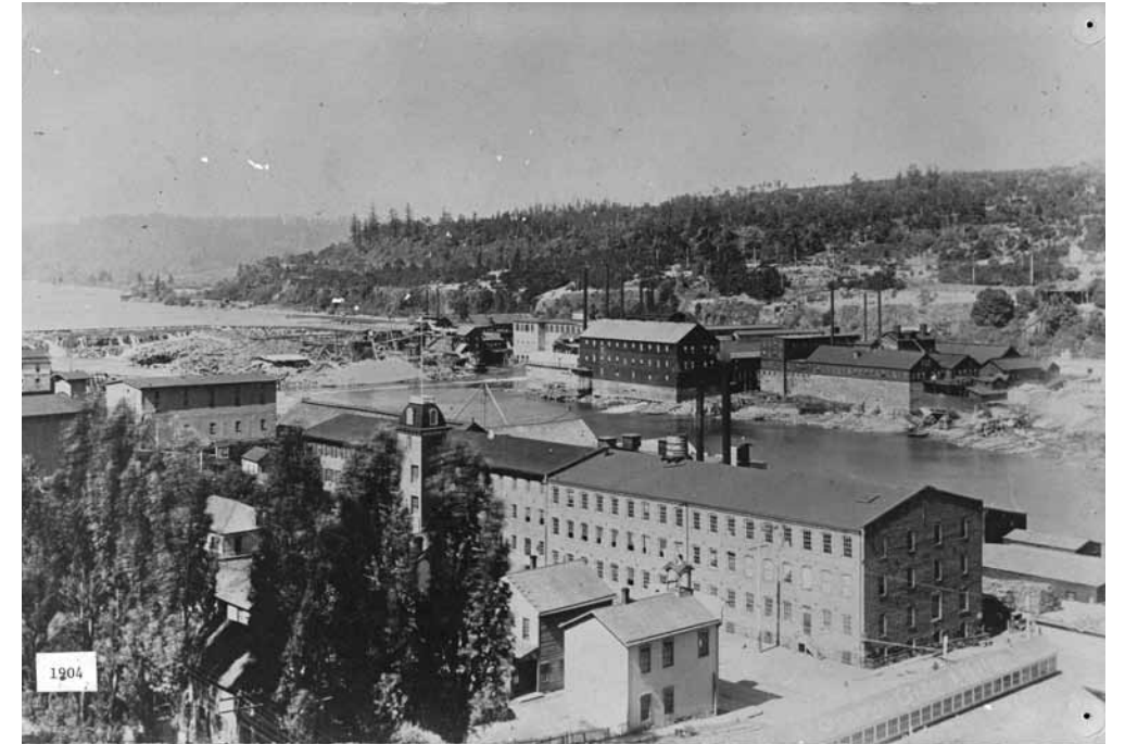
The foundations of the original Woolen Mill on Main Street (mill shown here in 1904) remain on site and could be incorporated into a new structure or open space.
