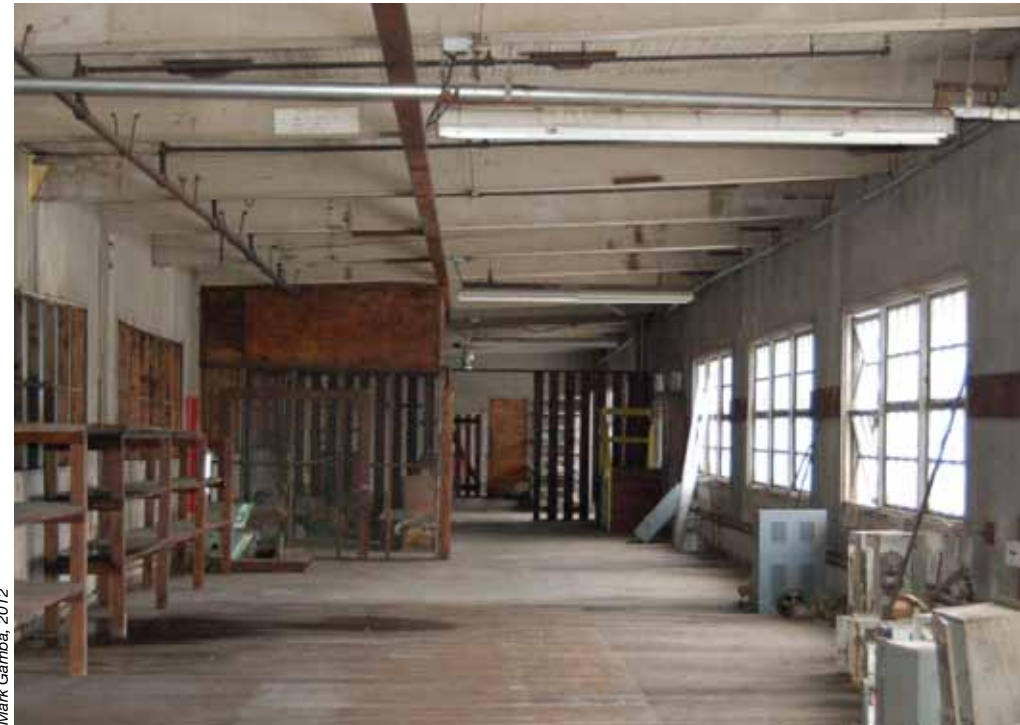
In addition to the massive concrete column and beam mill structures, wood framed buildings exist on site with exposed wood columns, beams, and roof trusses. A renovated Mill O could be a unique space with distinct character.
