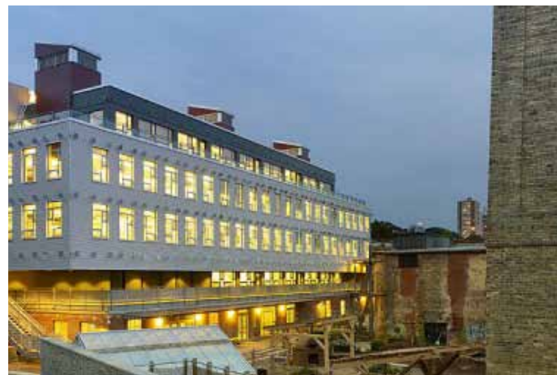
New construction at Evergreen Brickworks, a community center and non-profit organization in Toronto, Canada.
