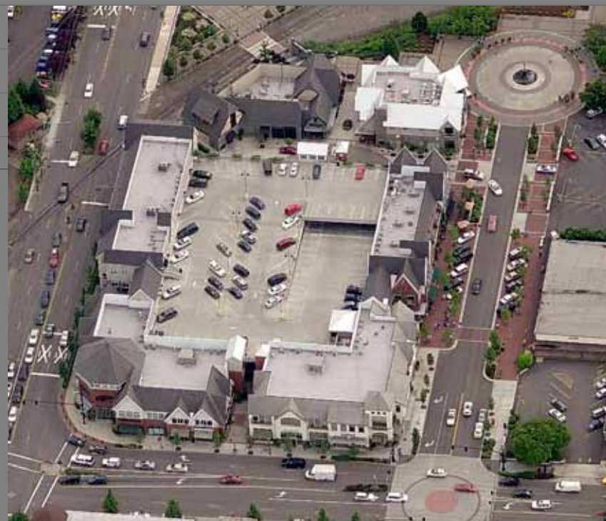
Lake View Village in Lake Oswego features 3 levels of public/private above-ground parking, hidden behind a liner of active, pedestrian-friendly mixed use.
