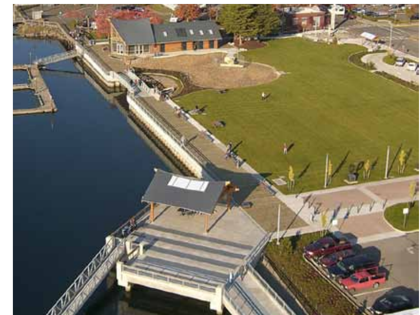
Percival Landing is a waterfront park in Olympia, built in phases over the last 30 years. The most recent phase, above, replaced a tank farm with open lawn, a waterfront walk and pavilions. With year-round activities, the park has attracted over $20 million in new investment in nearby blocks.
