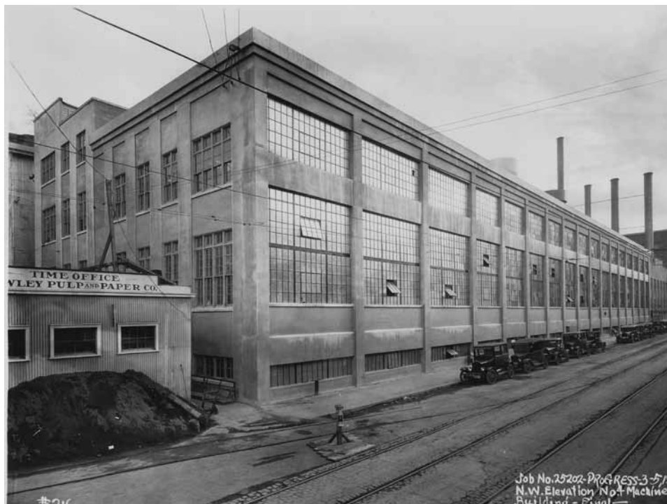
#4 Paper Machine has a strong presence and creates a well scaled urban street edge.
