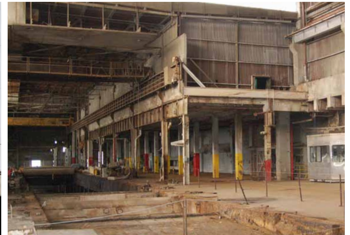
Expansive and flexible interior volume within the No. 4 Paper Machine Building.
