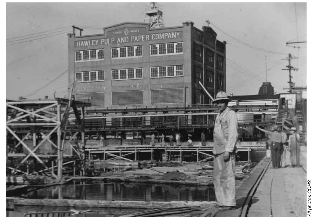
Hawley/#1 Paper Machine is a significant visual and historic icon and occupies a prominent position on the upper basin and at the south end of Main St.
