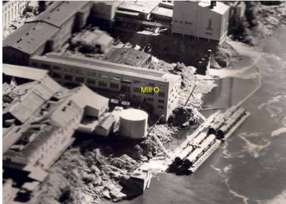
Mill O extends west from Main Street and the Woolen Mill in this 1955 photo.
