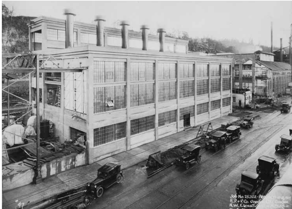
De-Ink Building exhibits a pure geometry that has been lost over a century of additions and renovations.
