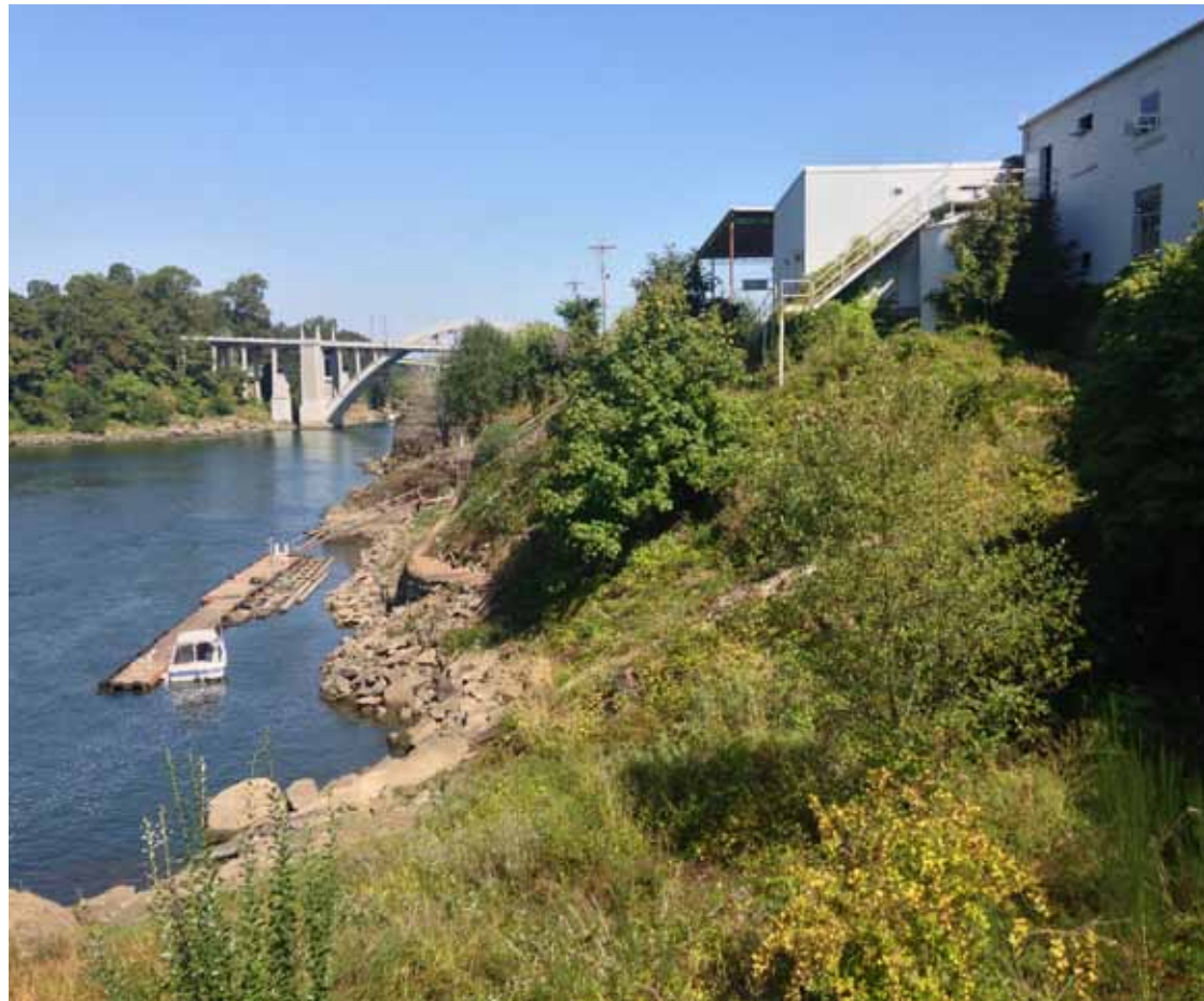
Degraded riverbank, overgrown with invasive species
