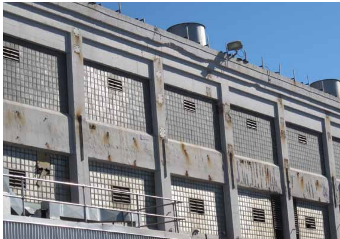
Even after the salvaging of materials, many of the existing mill structures retain an authentic industrial character and scale, with simple concrete forms, and can be repurposed.
