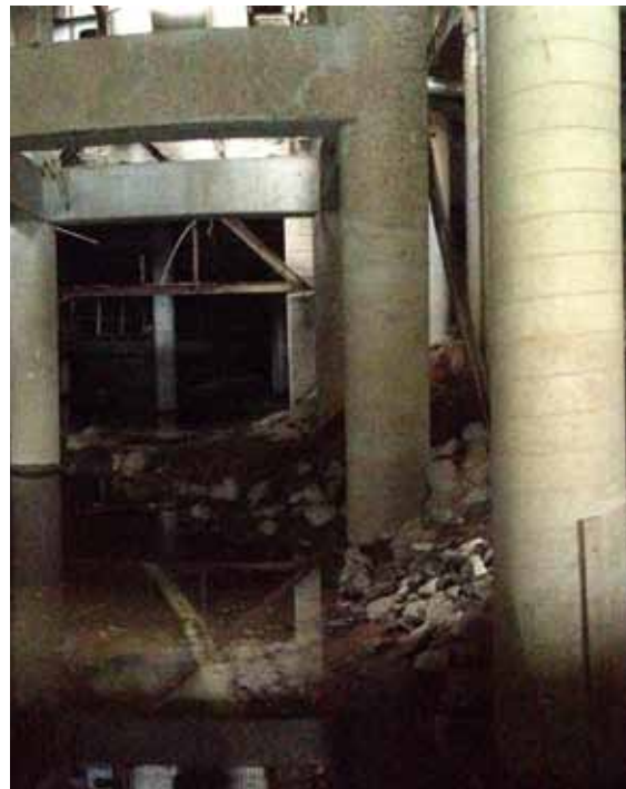
Former tailrace underneath Mill G
