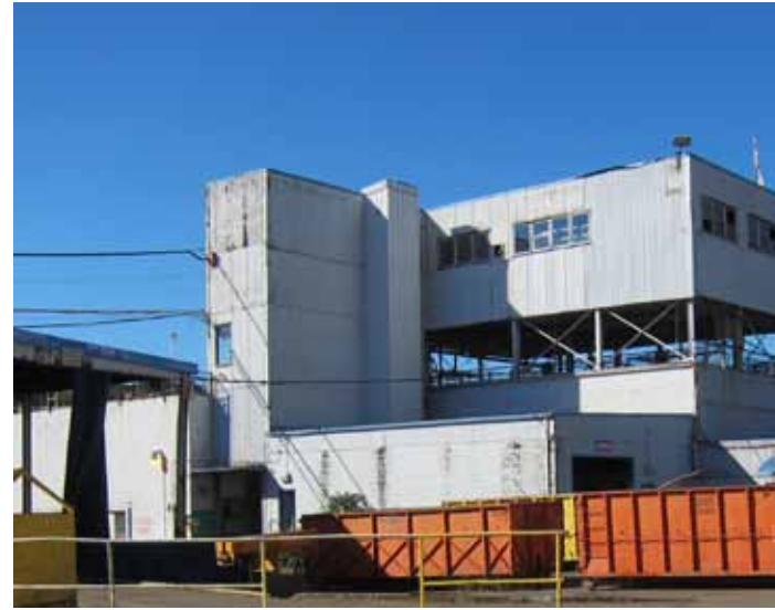
2. Water Filtration Plant
