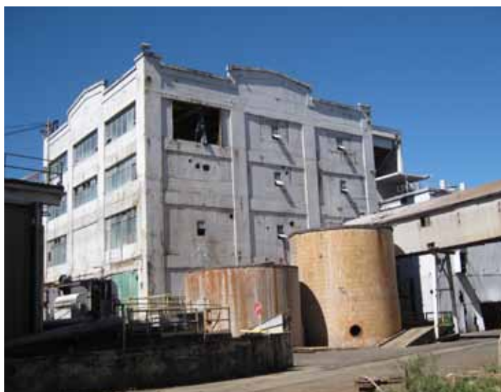
32. Hawley Office Building
