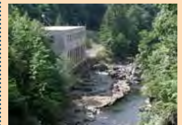
Bull Run River powerhouse
