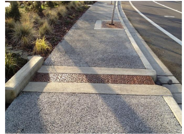
Caption: Sidewalk section of porous concrete alongside Warner-Milne Road in Oregon City.
