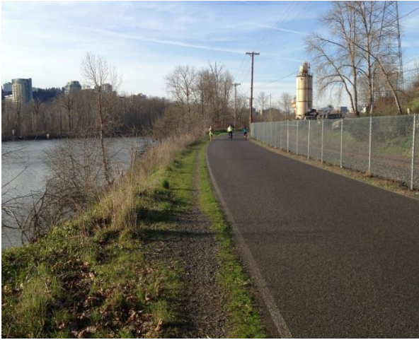
Caption: The Springwater Corridor along the Willamette River has visually permeable fencing that allows users to see what is coming around the bend. The presence of railroad tracks on one side and the Willamette River on the other side limits the shy distance for this section of the trail.
