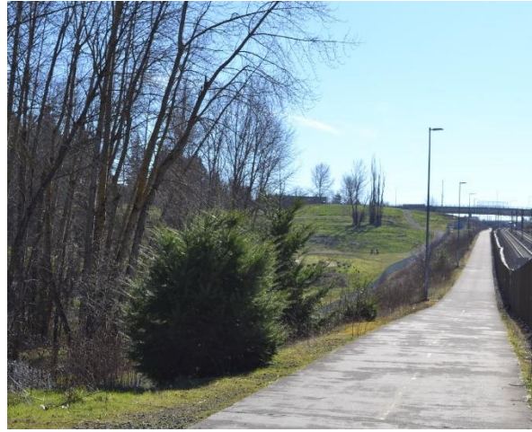
Caption: The I-205 Multi-Use Path parallels I-205 and the MAX Green Line through Multnomah and Clackamas counties. A striped yellow line delineates two-way traffic on the trail.
