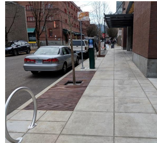
Caption: An oversized tree grate in the Pearl District in Portland maximizes soil volume over a typical street tree installation. Stormwater runoff from the adjacent sidewalk panels will flow into the tree opening. This installation could further be enhanced by providing root paths under the pavement or connecting to a similarly installed street tree planting and grate system to create a continuous trench.
