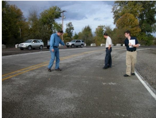
Caption: A roadway section of pervious asphalt.
