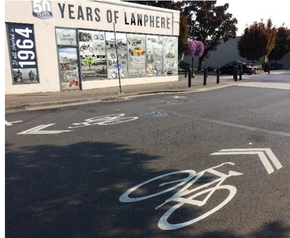
Caption: A shared lane on streets with low traffic, less than 1,500 vehicles a day, also known as a bicycle boulevard. Pavement markings and bike wayfinding alert drivers to expect bicyclists on the street and alert bicyclists to “take the lane.” This bicycle boulevard in downtown Beaverton provides access to businesses and services.
