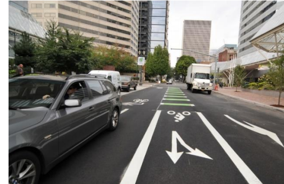
Caption: A standard bike lane, typically about 6 feet wide and immediately adjacent to motor vehicle travel lanes. This type of facility should not be used on streets with more than 3,000 motor vehicles a day and/or operating speeds greater than 30 miles per hour. This bike lane connects to Portland’s Waterfront Park.
