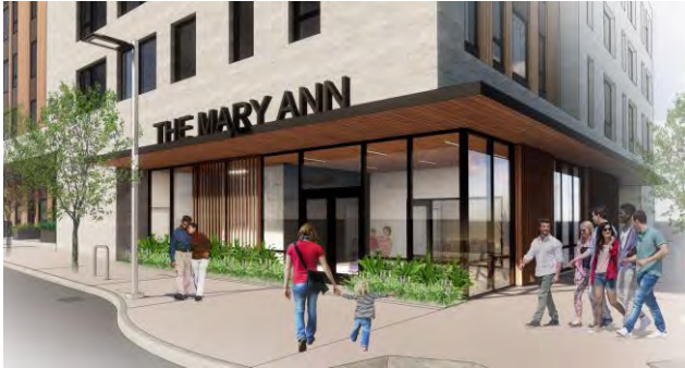
“The Mary Ann” Apartments | Downtown Beaverton City of Beaverton Total Units: 54 30% AMI Units: 11 Family Size Units: 29
