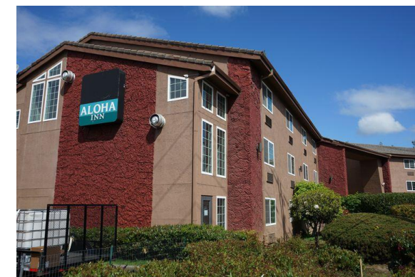
Aloha Inn, WA County
